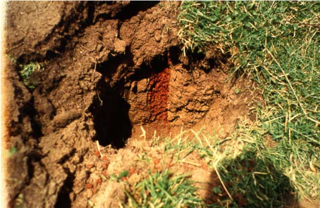
Figure 4. Gravel mole drain (slot filled with gravel)
